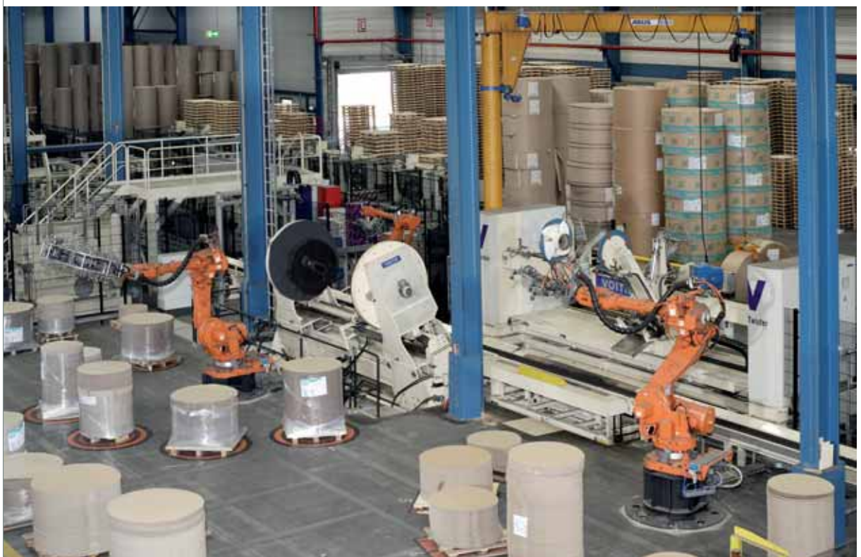
Robot-controlled twister packaging system in the Kehl mill
